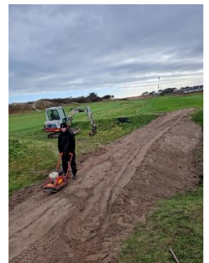
New walkway installation on 18
