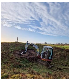
Sand scrape work at Barbers Pole
