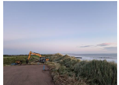
New 7 th tee during construction
